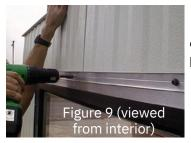
9. Anchor the head fin to the wall panel with self tapping screws (by Butler) through the pre-drilled holes in the head fin.
